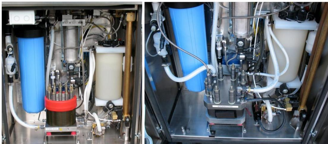
**Figure 4.** The HOGEN® electrolyzer with the original cell stack (L) and the Next Generation cell stack (R) installed
